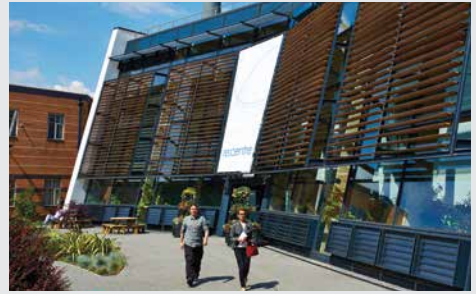
The University of Bradford's Bright Building, one of the UK's most sustainable buildings according to BREEAM, (Building Research Establishment Environmental Assessment Method).
